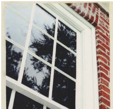
Fully restored window, 1819 Thomas Hickman house.
